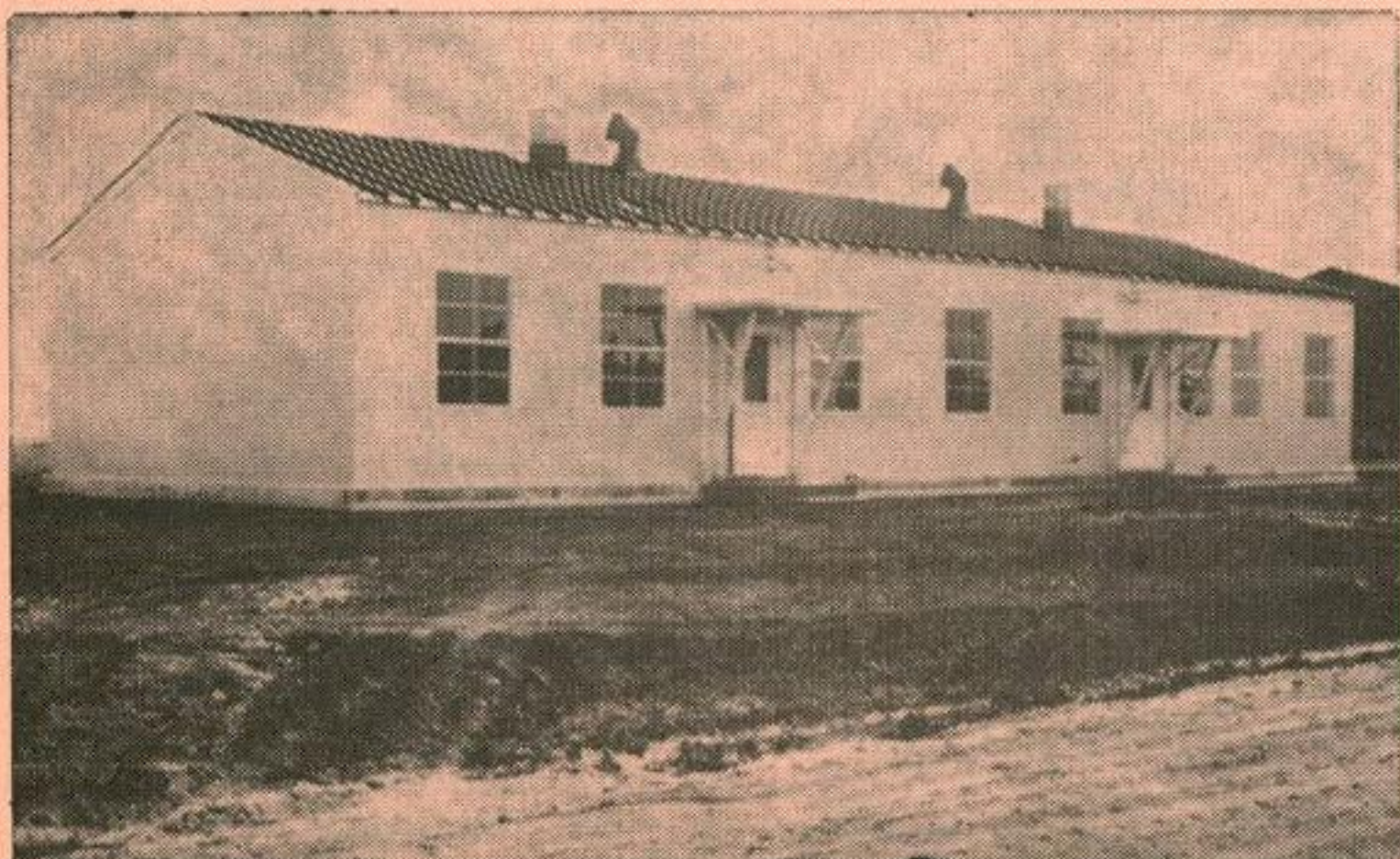
ONE OF THE STEELOX BUILDINGS used for Private Married Quarters, taken just after construction was finished.
