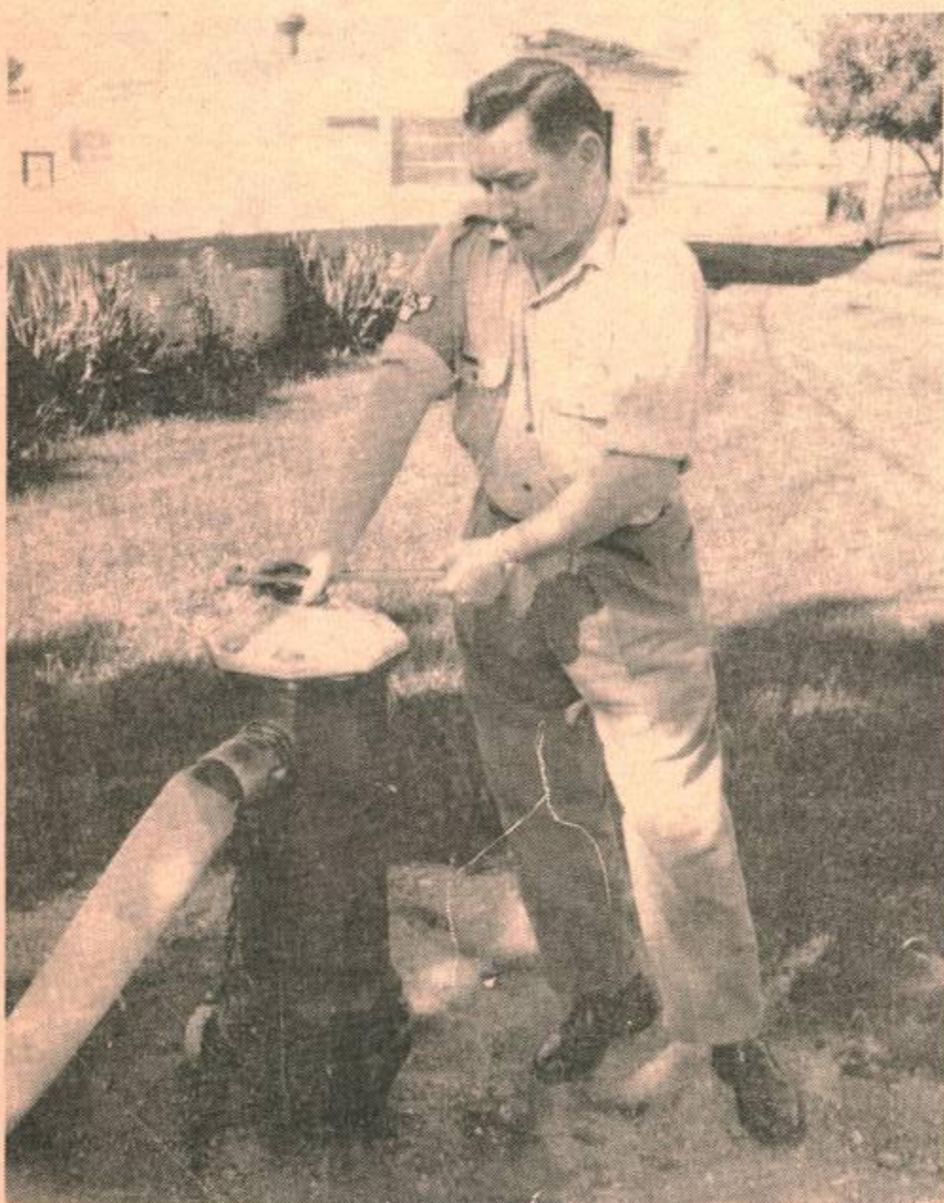
M/CPL. Ray Sisk ready to open a fire Hydrant
