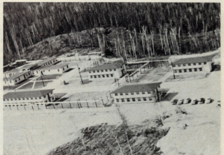
Aerial view of on-base quarter area. The mess hall and administration building are located in the main upper left building. The Operations site is located off to the left.
