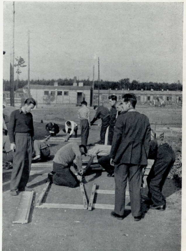
" THREE TIER BUNKS UNDER CONSTRUCTION "
