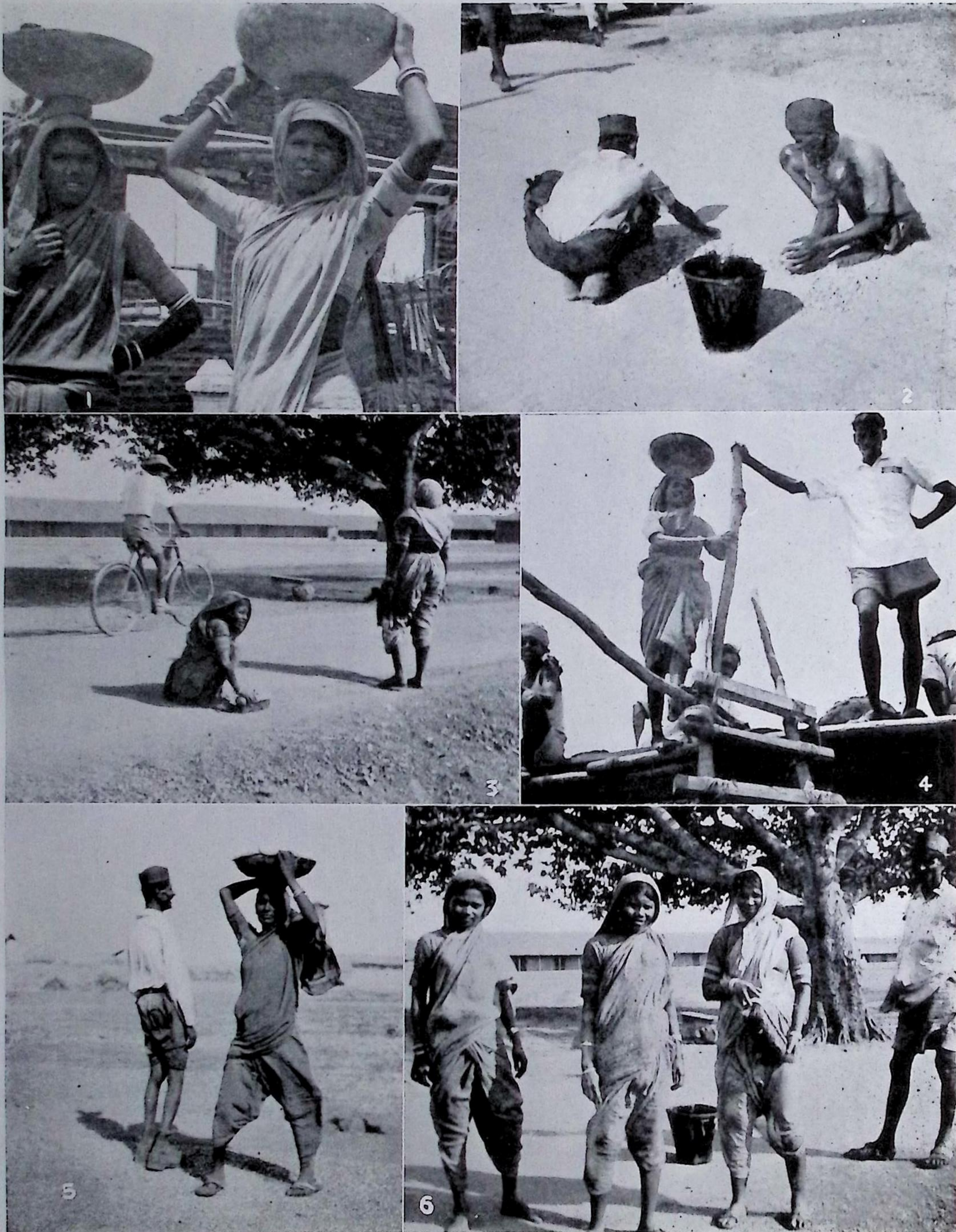
ROAD BUILDING NEAR POONA.—1. Women carrying crushed rock and tar. 2. Men placing the crushed rock in roadway mopped with tar. 3. Coolie women sweeping the completed roadway. 4. Construction is done by men, while women supply materials. 5. Coolie woman ready to scatter crushed rock over tarred road surface. 6. Coolie women pose for cameraman.
