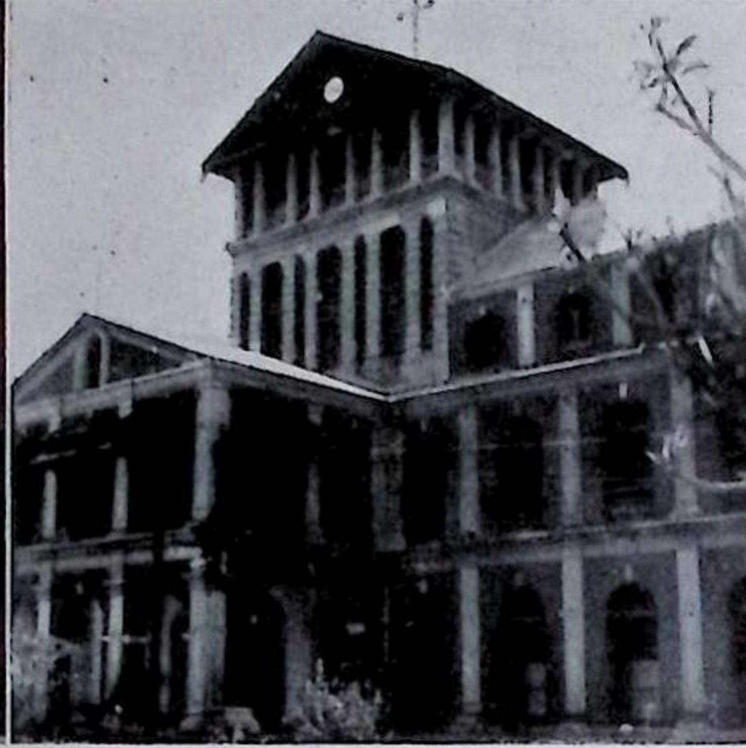
Main Hospital Building at the Leper Asylum
