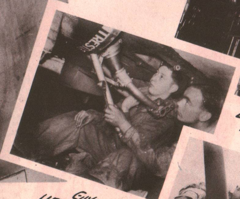
GIVING THE LIFTING PROBLEM THE ONCE OVER
