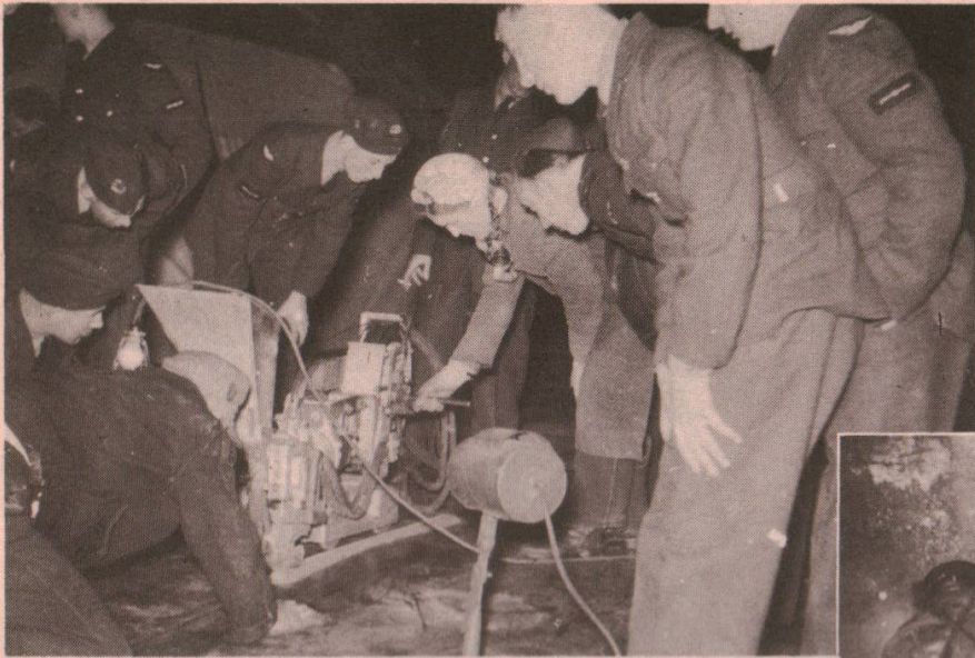
INSPECTING THE UNION WELDING MACHINE
