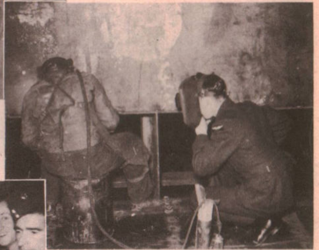
WATCHING A WELDER
