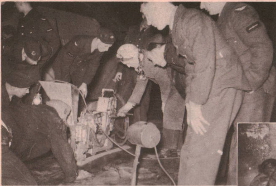
INSPECTING THE UNION WELDING MACHINE
