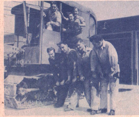
Tightening the tracks on a crane.
