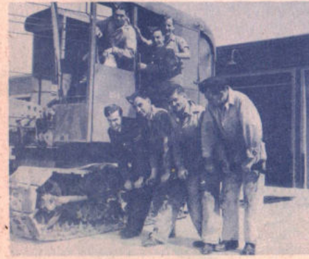
Tightening the tracks on a crane.
